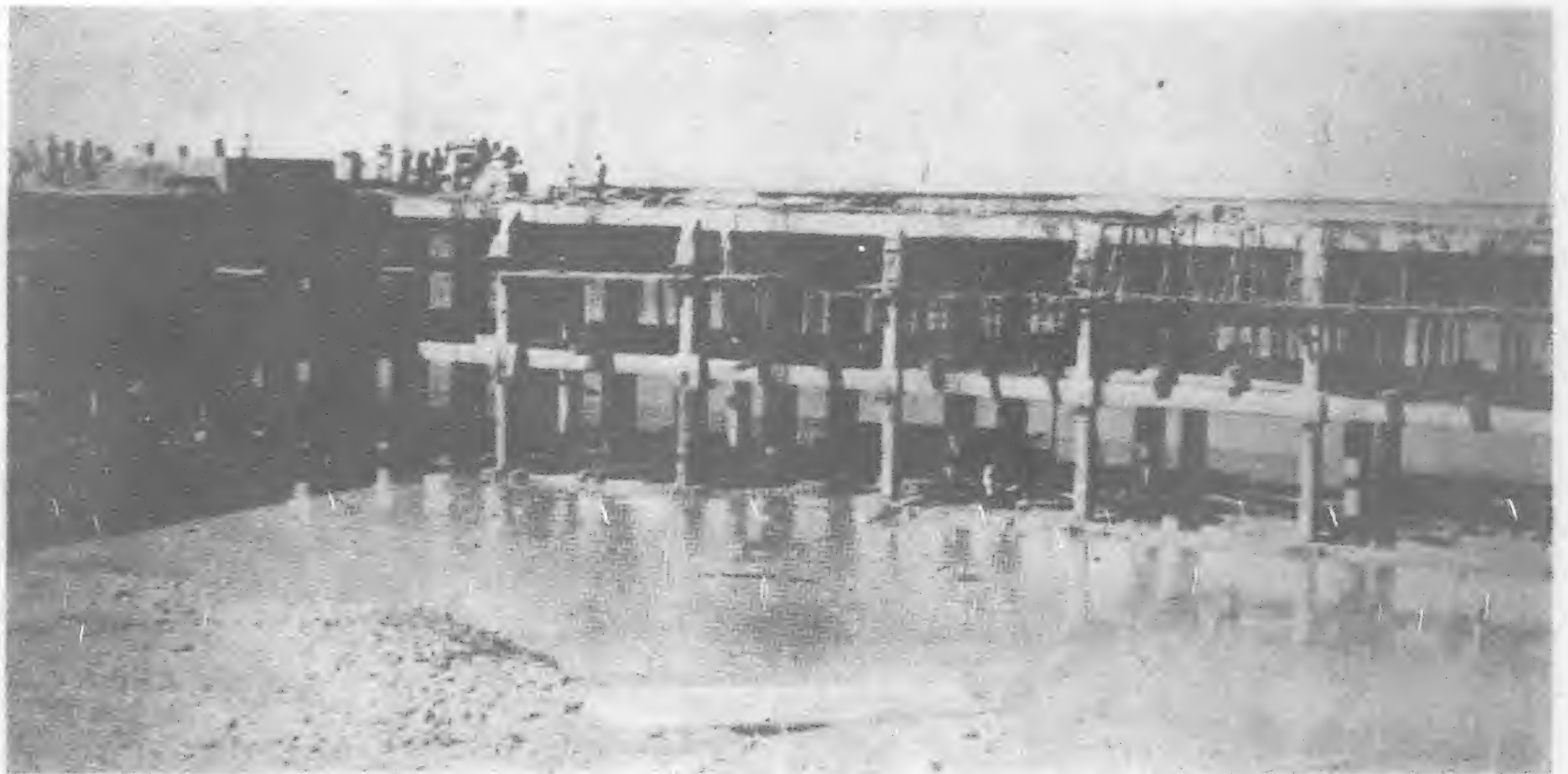
Main jetty between road approaches 1 and 2, January 14, 1936
